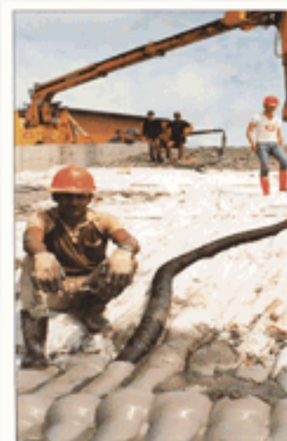
Injection of concrete
