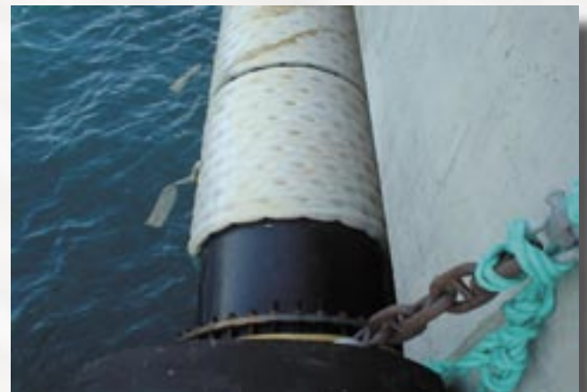
FlexiTex used as ballast on pipes
